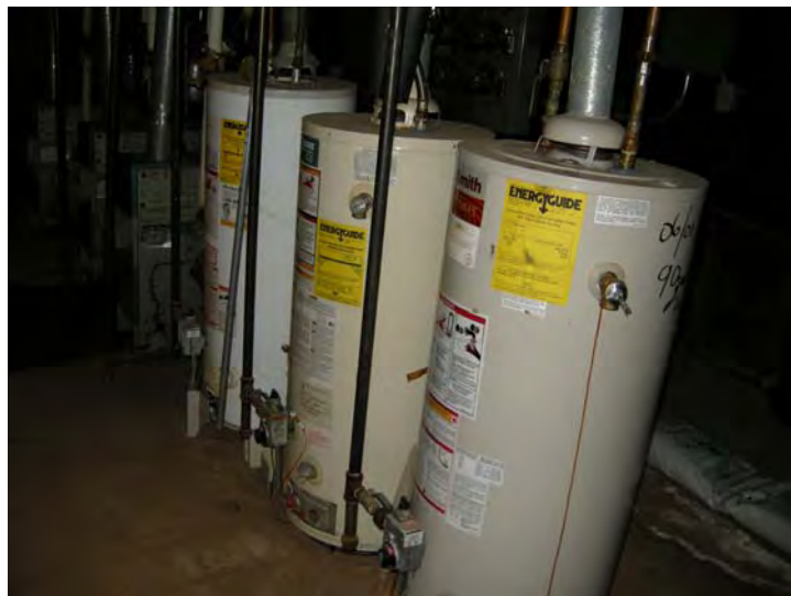
Typical array of domestic hot water heaters
