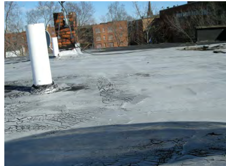
Typical roof section. Ward and Affleck roof coverings are reported to be similar.
