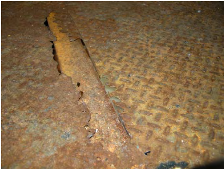
Example of rusted through deck plating at the rear deck and stair assembly of Affleck Street
