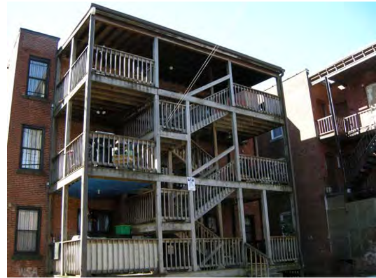
The wood deck and stair assembly at Ward Street
