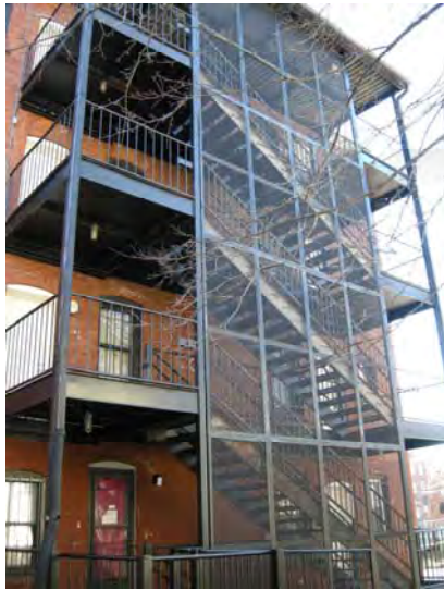
The rear elevation and metal deck and stair assembly at Affleck Street
