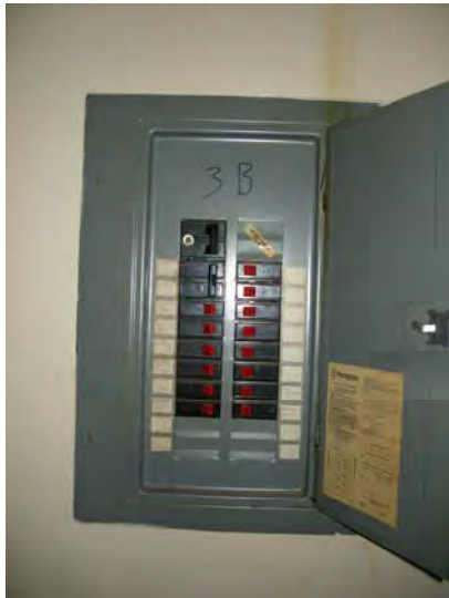
Typical circuit breaker panel
